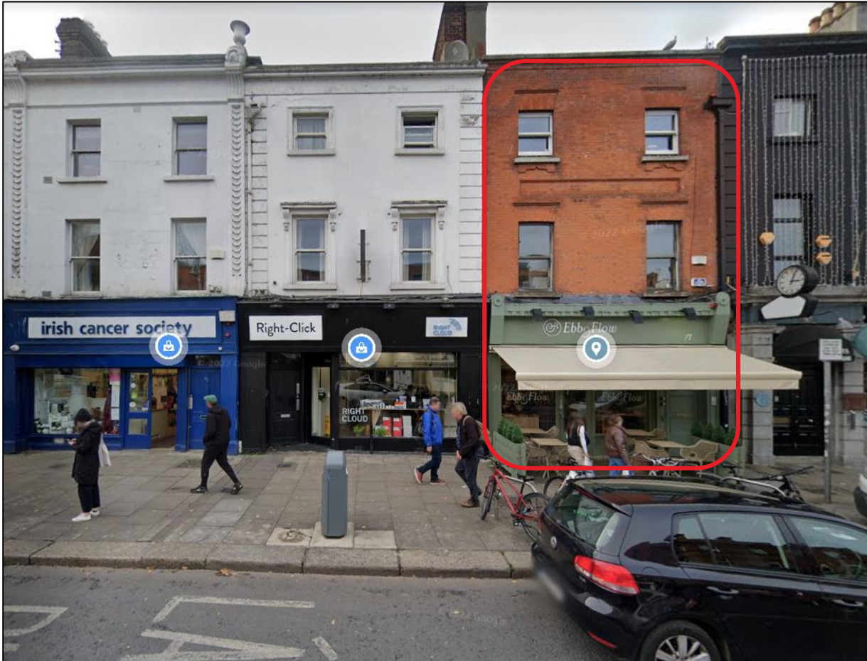
Figure 3.2.5 Existing frontage of 71 Camden Street Lower (Image source: Google)
