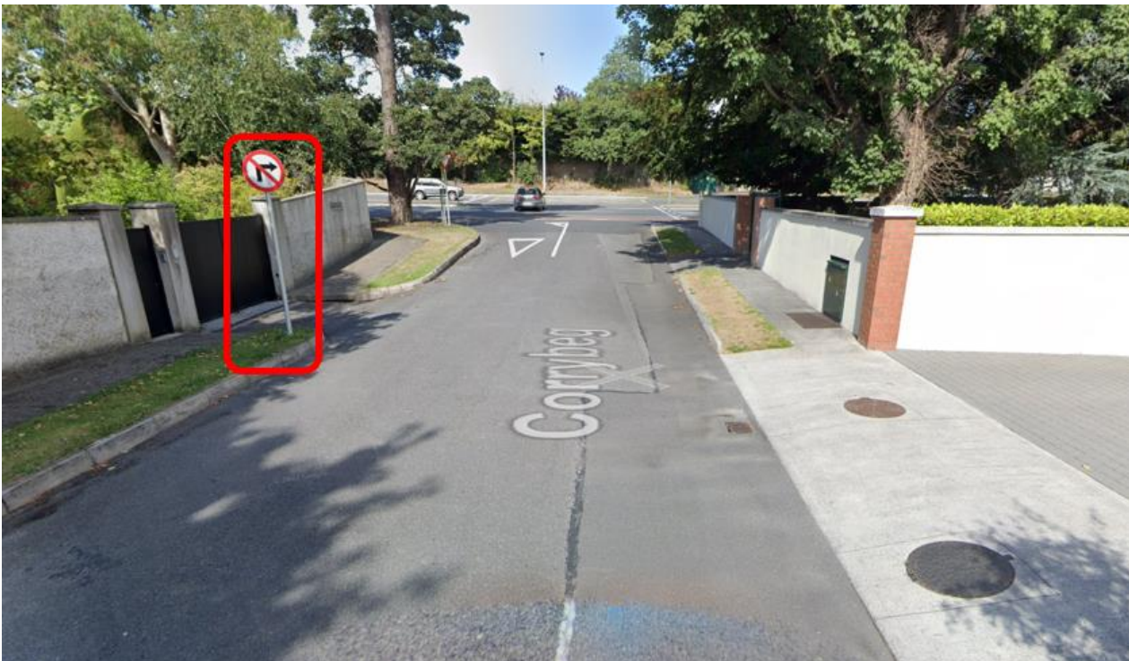
Figure 3.63.24 Existing no right turn sign on Corrybeg
