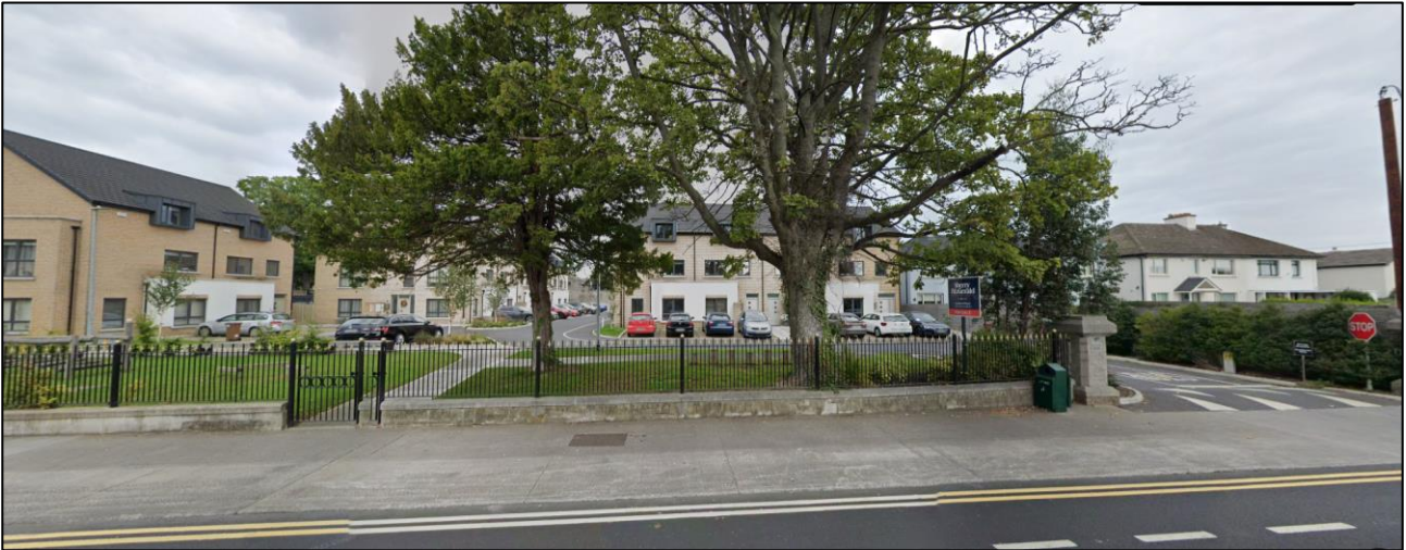
Figure 3.5.5 Existing frontage of Ashfield Place (Image source: Google)
