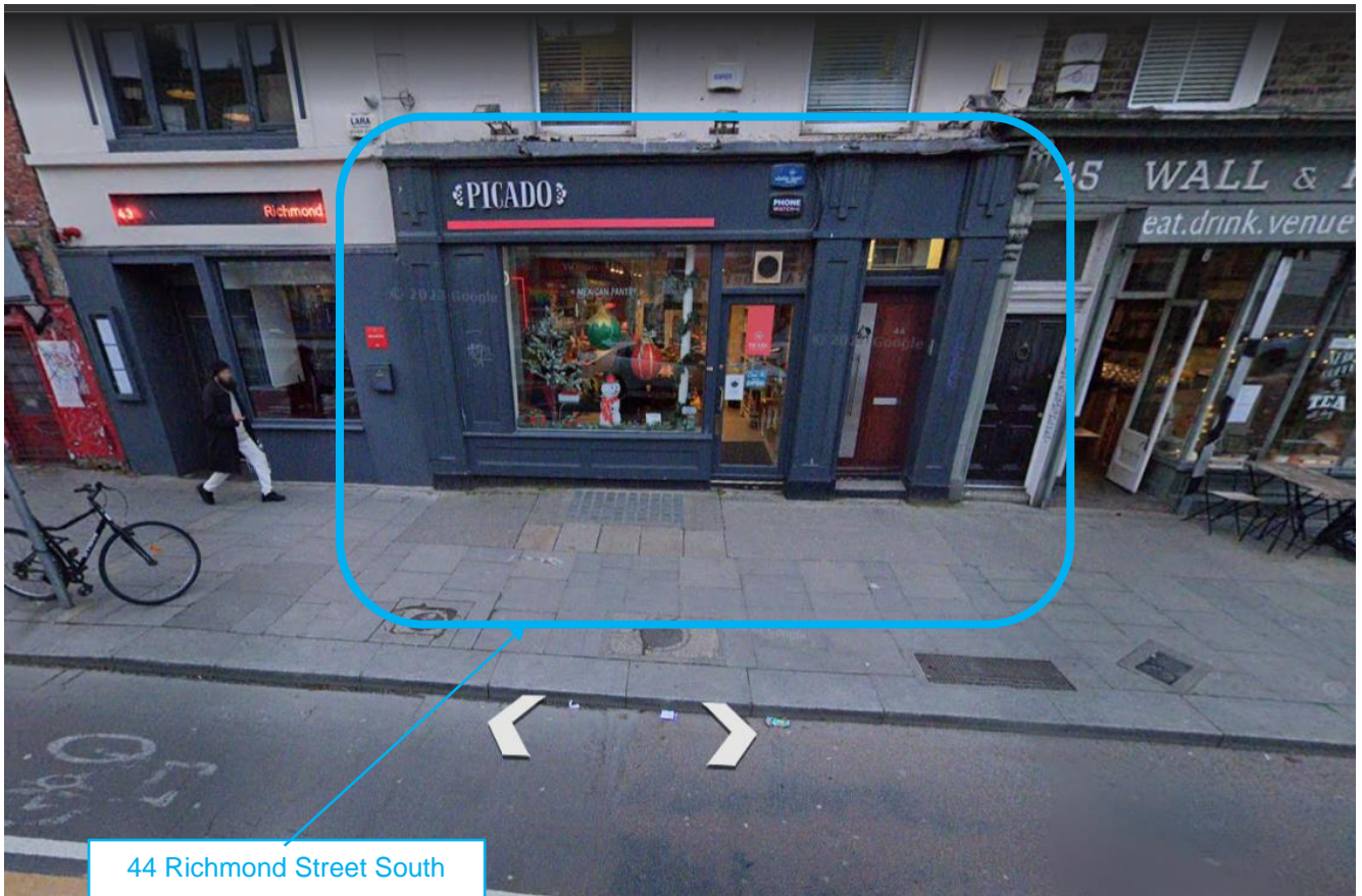
Figure 3.26.5 Existing view of 44 Richmond Street South (Image source: Google)
