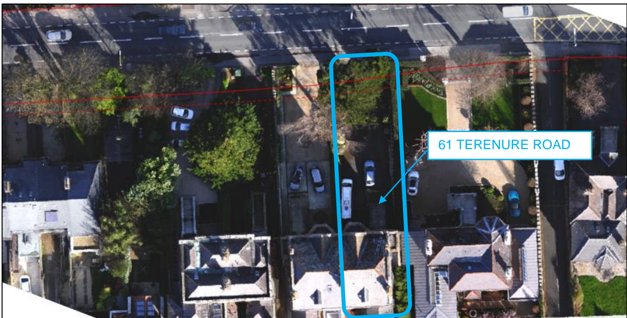
Figure 3.44.4 Proposed Land Acquisition lines at laneway adjacent to 61 Terenure Road East The existing property frontage is shown in Figure 3.44.5.
